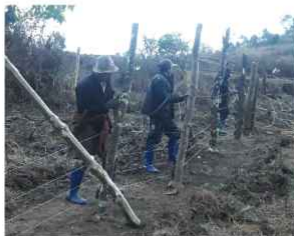
Electric Fencing at Lhuentse
