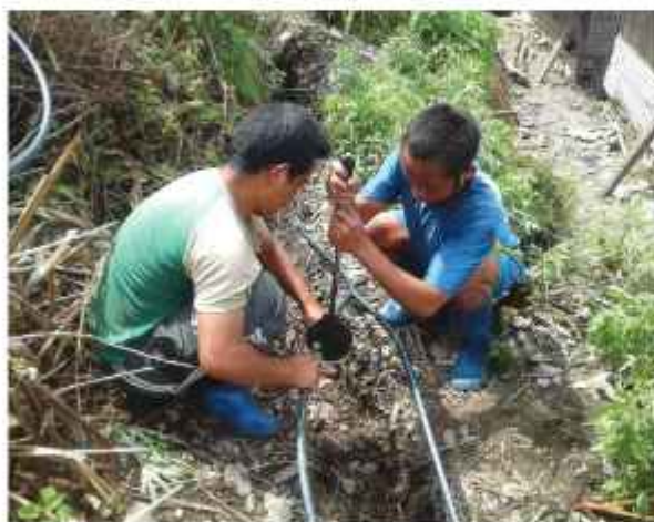
Fixing Water Pipeline at Samtse
